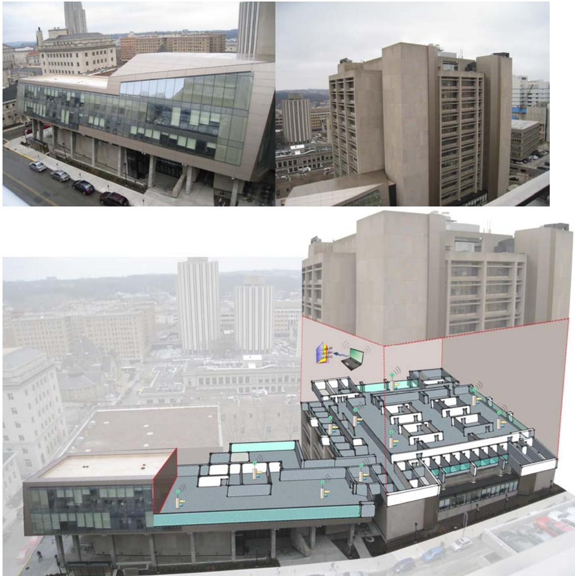
Figure A1 - Photos of case study building. Upper Left - MCSI addition (constructed 2009). Upper Right - Benedum Hall tower (constructed 1971; renovated 2009). Lower - cutaway view showing MCSI addition and renovation of tower 2 nd floor.
