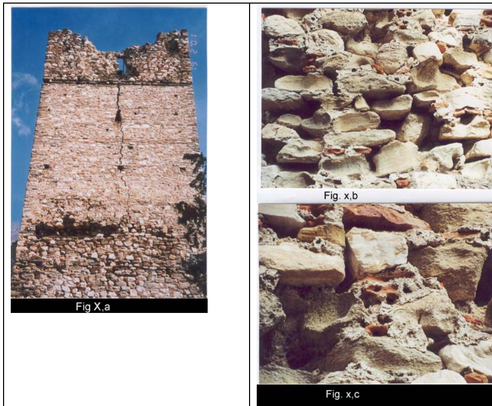
Fig. 3.7.1 a. Tower of the castle of Serbia (N. Greece, 11 th century) suffering from erosion; b/c. details of the eroded lime mortar.
