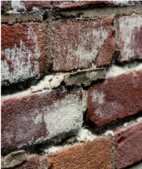
Fig. 3.2.1 As a result of salt crystallisation at the interface between bedding and pointing mortar the pointing has been forced out.
