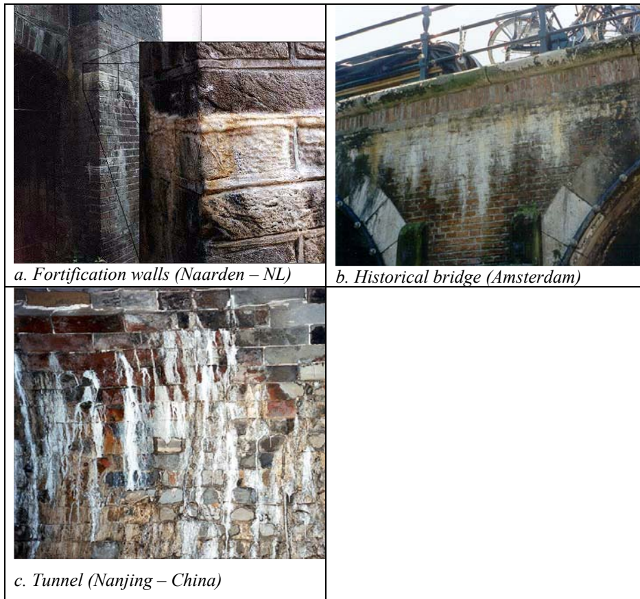
Fig. 3.6.1 Examples of encrustations. Especially in the case of the wall belonging to the fortification (a) the hard and glassy structure, which is difficult to remove, is clearly visible. Leaching may sometimes lead to the formation of stalactites as the Nanjing example (c) is showing.
