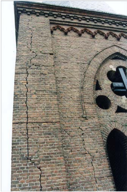
Fig.3.3.1 Wide (vertical and also horizontal) cracks, on the first sight looking like structural cracks, were found to be caused by swelling compounds in the inner part of the masonry.
