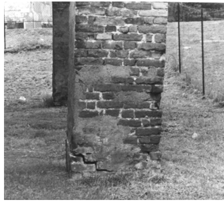
Fig. 3.14.2 Cracks in the mortar joints
