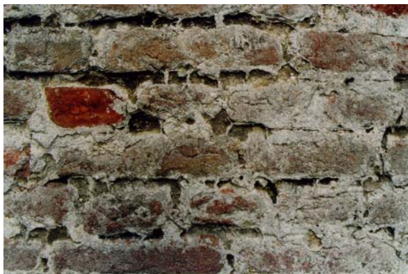
Fig. 3.7.2 Detail of eroded lime mortar of an old town wall.
