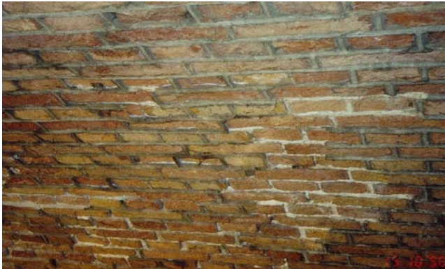
Fig. 3.3.2 Damage in the passage(way) of a historical arch bridge: spalling of brick and pointing is pushed out.
