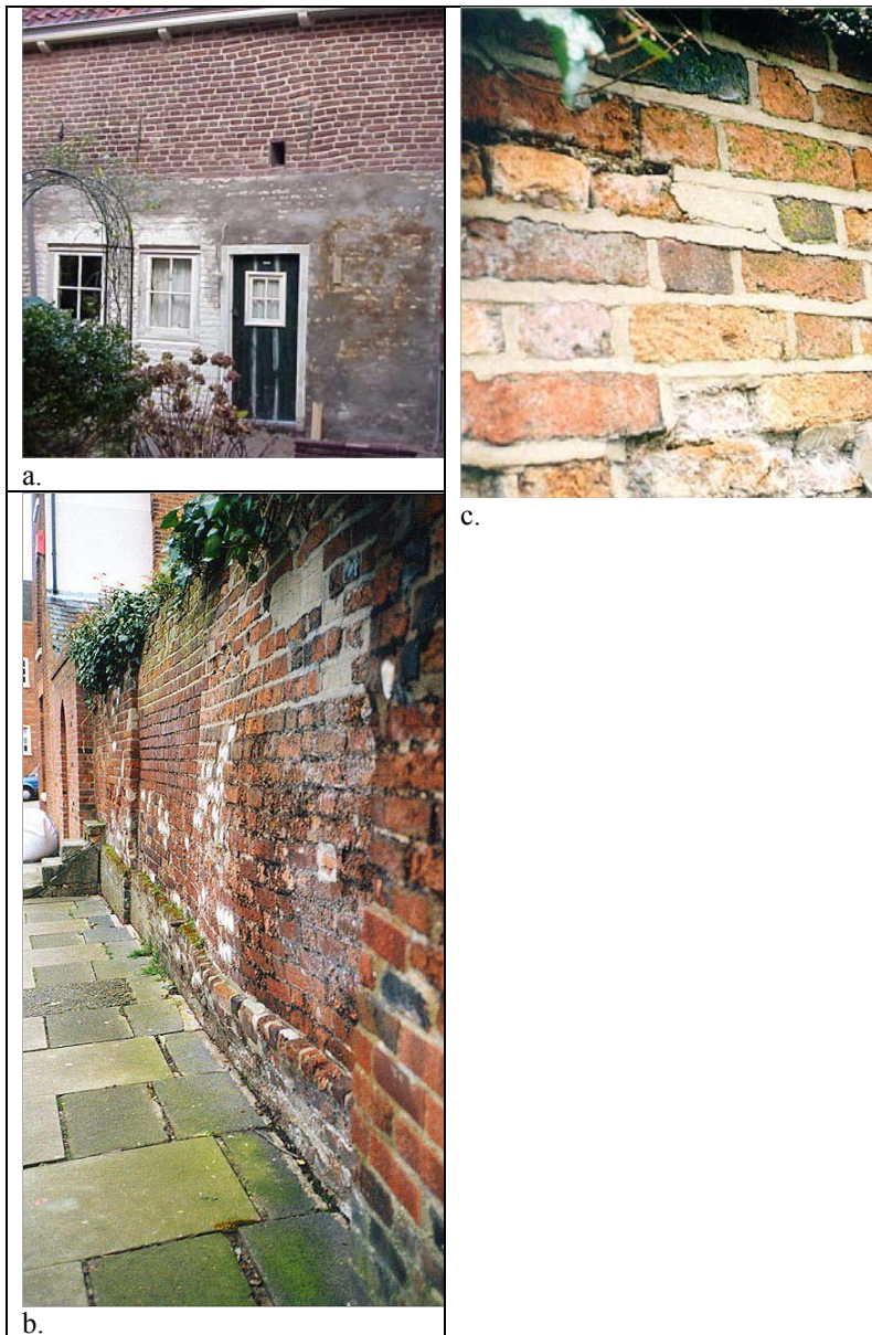
Fig. 3.11.2 Examples of deformation in lime mortars. (a). Setting of masonry in a façade. (b). Bulging of a garden wall. (c.) Detachment of cement re-pointing in the wall shown in b., not following the deformation.
