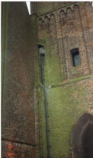
Fig. 3.10.2 Growth of algae caused by to low capacity of gutters and downpipe.
