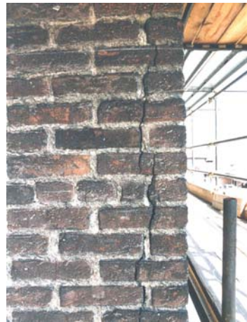
Fig. 3.13.6 Cracks at the corner of the bell tower.
