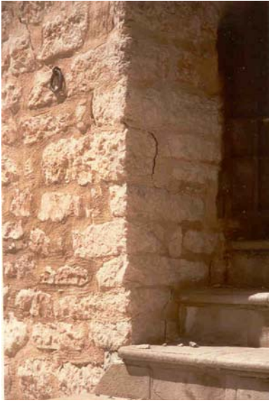
Fig. 3.15.1 Diagonal damage, running through Horizontal and vertical joints
