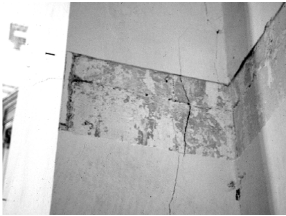
Fig. 3.13.11 Example of creep damage in the pillars of the Church of SS. Annunziata, Ispica, Sicily. It is clear that the cracks on the putty lime plaster are thinner than the ones underneath it. In fact the plaster is also detached as visible in the upper part on the right of this photograph.
