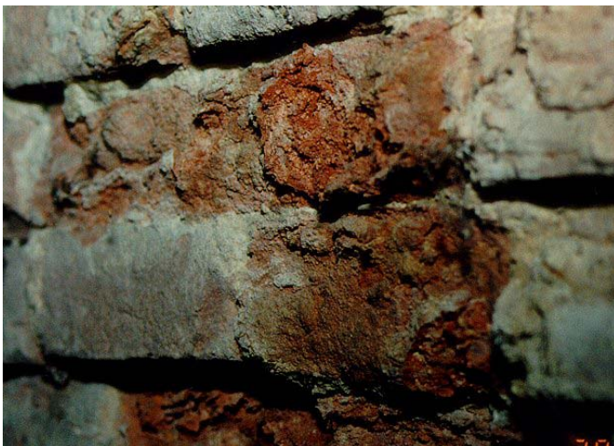
Fig. 3.5.2 Crumbling and bursting of the brick inside the windmill.
