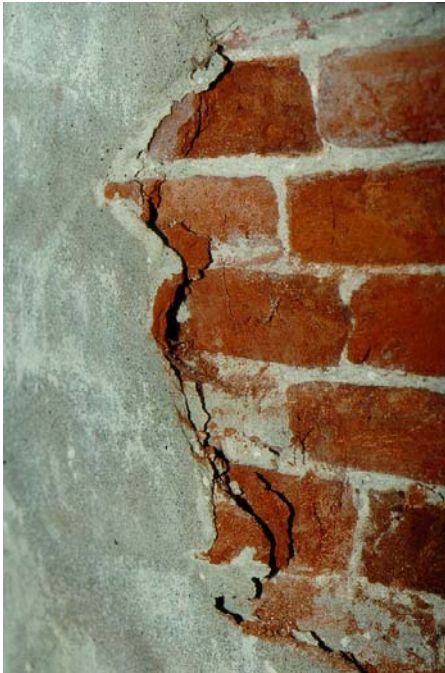
Fig. 3.5.1 Exfoliation (layering) of plaster and masonry inside the windmill.
