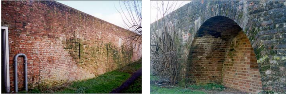
Fig. 3.10.1 Examples of algae growth on an old city wall.
