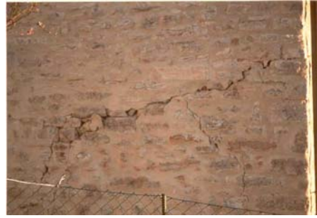
Fig. 3.15.2 Diagonal cracks involving mortar joints and stones
