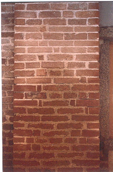
Fig. 3.12.1 Wet zone at lower part of one of the columns.
