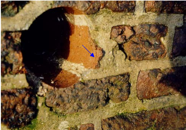
Fig. 3.3.3 Start of damage visible in the hole left by the drilled core (see arrow for location): a layer of the brick begins to detach, the bedding mortar shows loss of cohesion.
