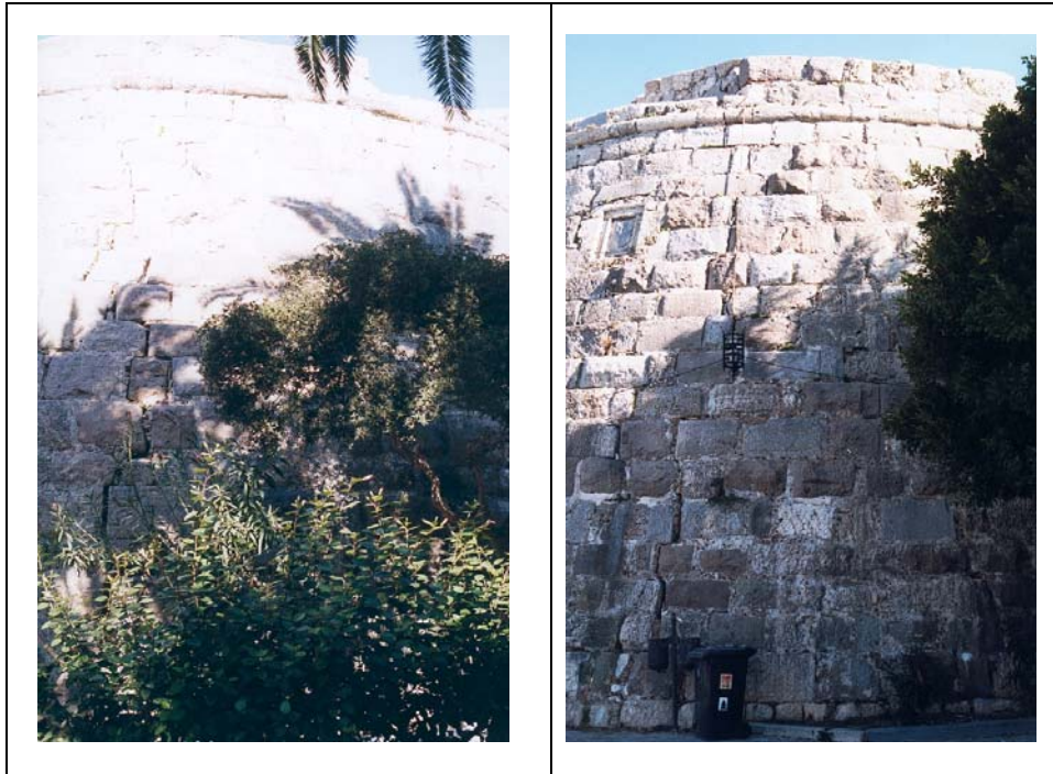
Fig. 3.13.2 Vertical cracks located at two different areas of the bastion
