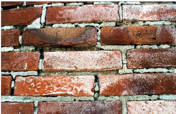
Fig. 3.8.1 Decay of pointing mortar (voids) due to sea salt action. Notice that the decay starts at the interface between brick and mortar.
