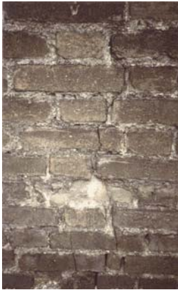
Fig. 3.13.4 Cracks passing through in brick masonry of a bell tower.
