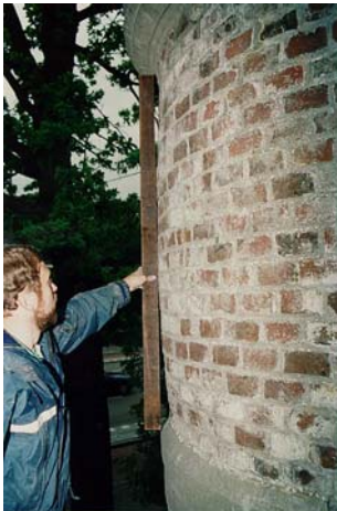
Fig. 3.1.1 Bulging of masonry. This part of the wall was already furnished with new pointing.
