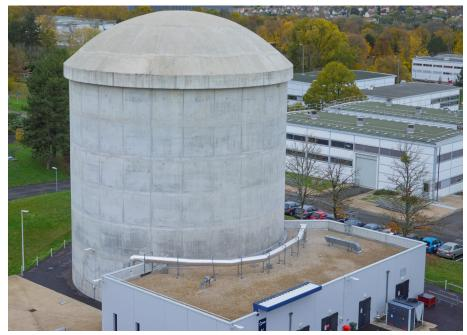
VERCORS A double wall containment of H:30m & Ø:16m. 5000 t of concrete 1 year of construction 1 auxiliary building (ventilation, heating, data) 500 sensors 2 km of fiber optic cables
