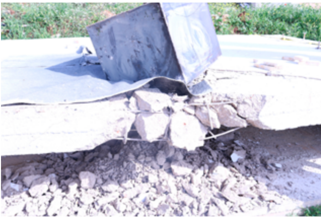
Impact of a 600 kg Reinforced Concrete (RC) block on a Post-Tensioned (PT) Slab ©Ali Jahami, Mohammed Sonebi
