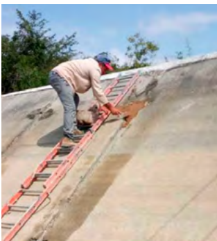
Placing the mortar in the channel joints ©TC282-CCL
