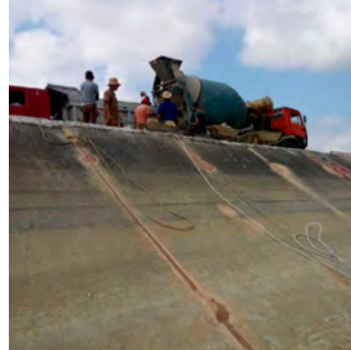
Channel with joints repaired ©TC282-CCL
