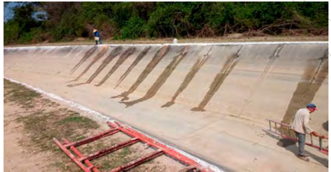
Moistening the joints ©TC282-CCL
