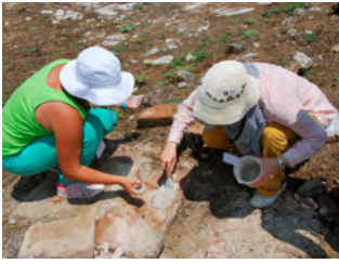
On-site application of lime-based mortars ©Laboratory of Building Materials, AUTH
