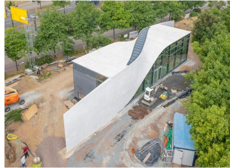
Carbon reinforced concrete house CUBE in Dresden, Germany. Image courtesy of S. Gröschel.
