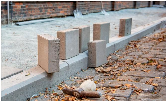
Image of demo-site in the city of Ghent, Belgium, showing a footpath of carbonation hardened pavers containing no Portland cement, only milled steel slag and aggregates. Image courtesy of VITO.
