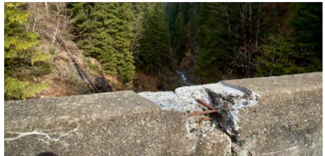
Damage produced by the corrosion of the steel reinforcement in concrete elements. Images courtesy of U. Angst.
