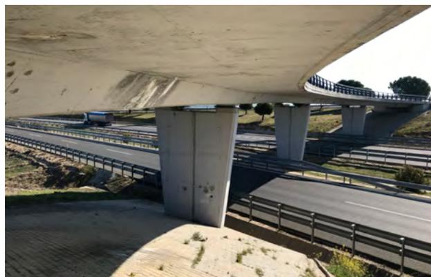
Corrosion damage in structural elements of transport infrastructure made of reinforced concrete. Images courtesy of C. Andrade.
