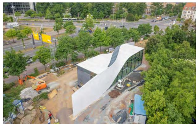
Carbon reinforced concrete house CUBE in Dresden, Germany. Image courtesy of S. Gröschel.
