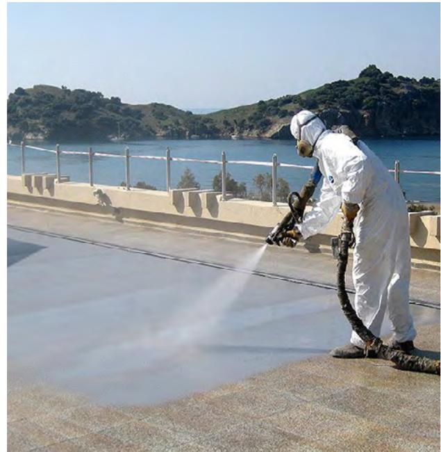
Technician spraying a waterproofing organic coating layer on a concrete roof. Image courtesy of Creamer Media.
