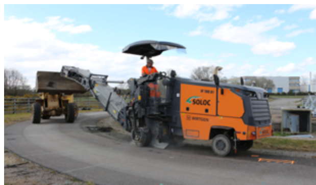
Extraction of old pavement containing alternative materials, shared through TC APS labs to assess their recyclability. Image courtesy of E. Chailleux.
