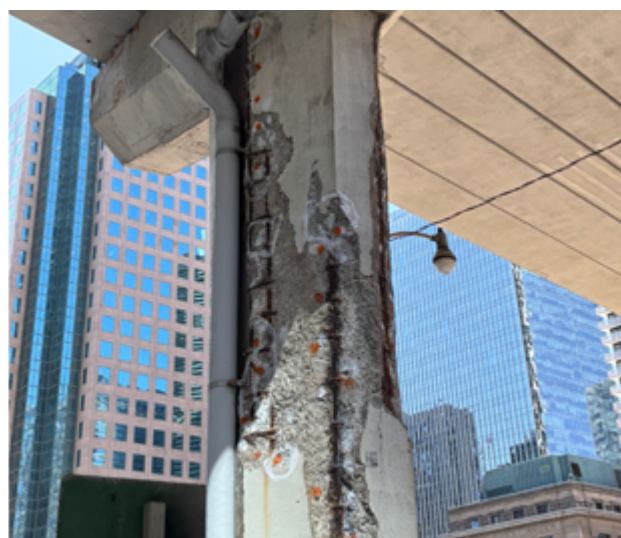
Advanced corrosion of reinforced concrete structural elements (column and slab). Image courtesy of U. Angst.
