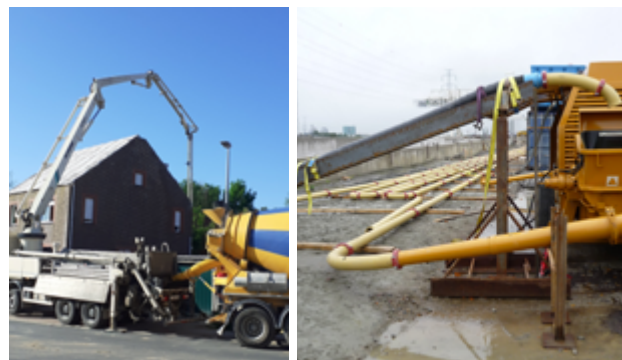
On the left: concrete pumping on a small construction site. On the right: large-scale concrete pump test on a major construction site. Image courtesy of G. De Schutter.
