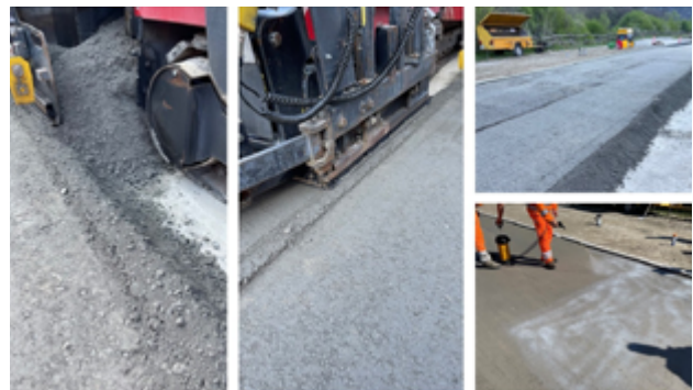
A trial along a roadway with RCC and a replacement of natural aggregates with RAP (reclaimed asphalt pavement 0-22 mm) of 20%. Image courtesy of C. Paglia.
