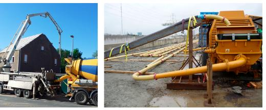
Concrete pumping on a small construction site and large-scale concrete pump test on a major construction site. Image courtesy of G. De Schutter.
