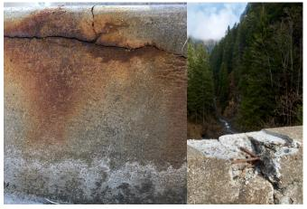
Damage produced by the corrosion of the steel reinforcement in concrete elements. Images courtesy of U. Angst.
