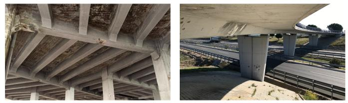
Corrosion damage in structural elements of transport infrastructure made of reinforced concrete. Images courtesy of C. Andrade.
