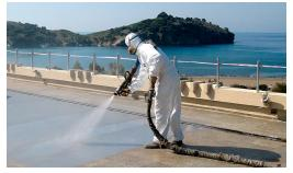
Technician spraying a waterproofing organic coating layer on a concrete roof. Image courtesy of Creamer Media.
