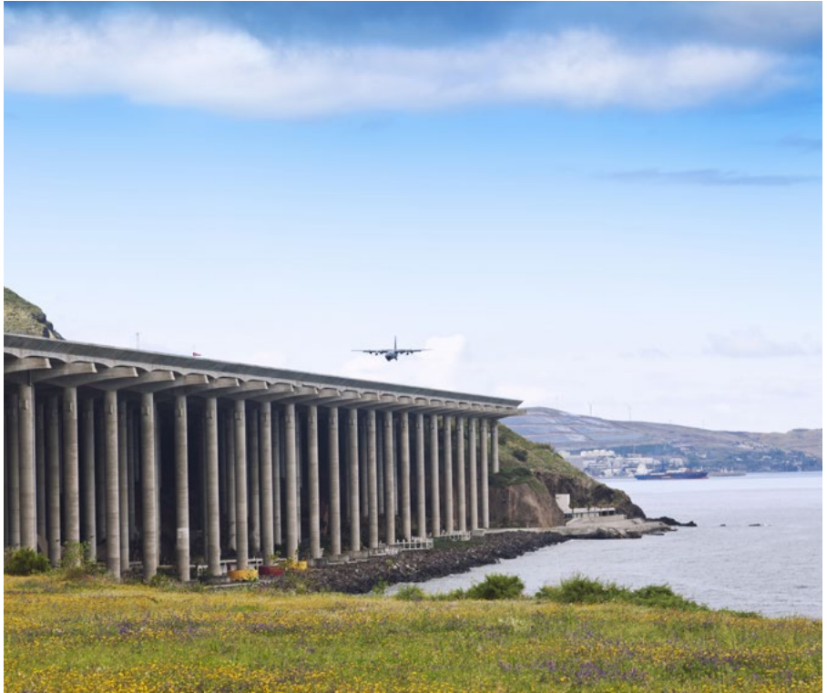
Madeira Airport to be visited in the technical tour.
