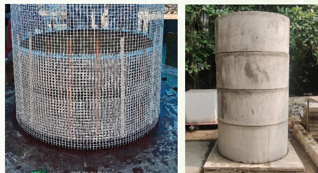
Circular sewage tank with TRC - at IIT Madras
