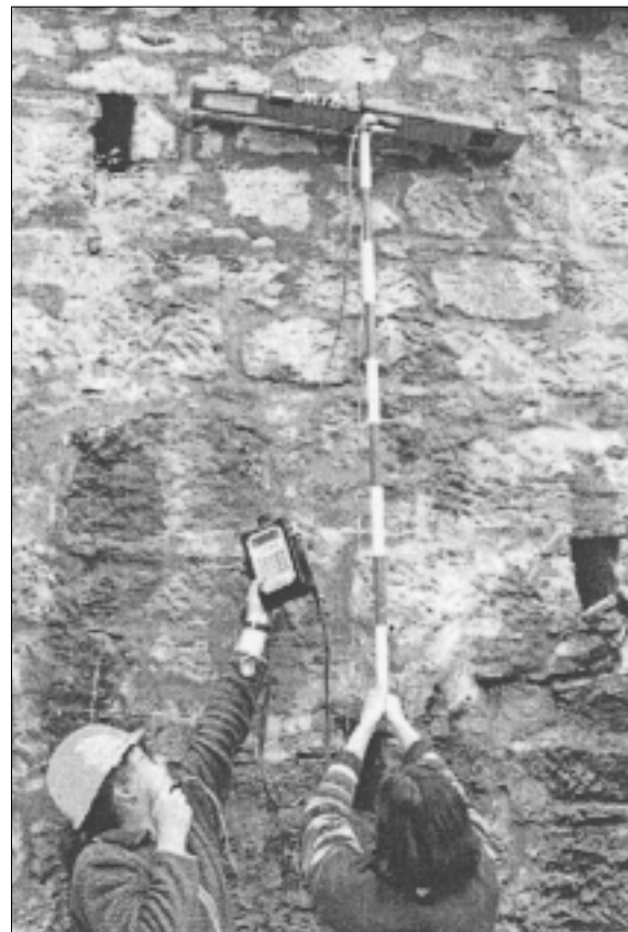
Fig. 2 – In situ conductivity data collection on stone masonry structure [6].
