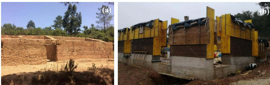
Figure 1: Rammed earth building located in Aljezur, Algarve: (a) old building (July 2021), photograph by Catarina Pereira; (b) new building under construction (December 2021), photograph by Bruno Coutinho
