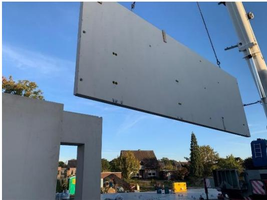
Figure 9: Prefabricated concrete elements “Büscher wall” from masonry rubble [11]
