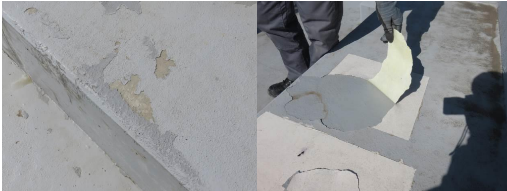
Figure 5: Surface coating deterioration (spalling, peeling...)
