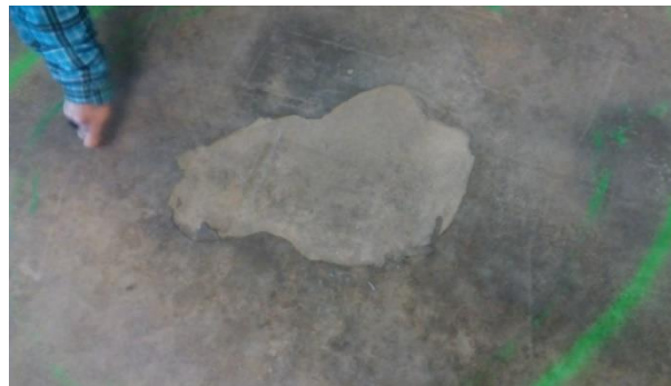
Figure 9: Surface coating spalling
