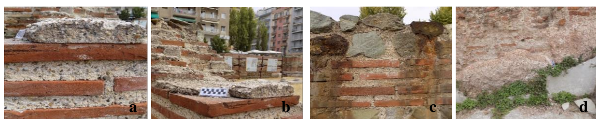
Figure 9 Deterioration phenomena of the repaired structures. a. microcracking, b. black crust, c. oxidation products, d. biological growth
