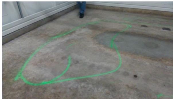
Figure 10: Surface coating spalling
