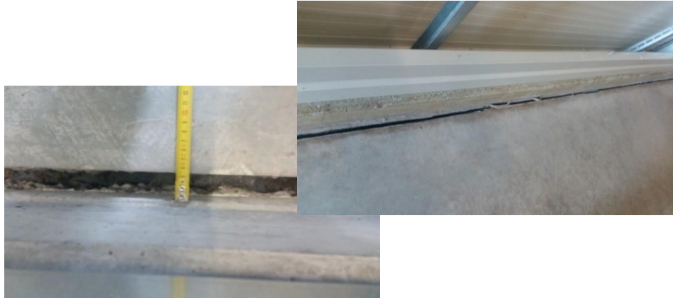
Figure 11: Joint gap at slab-beam connection
