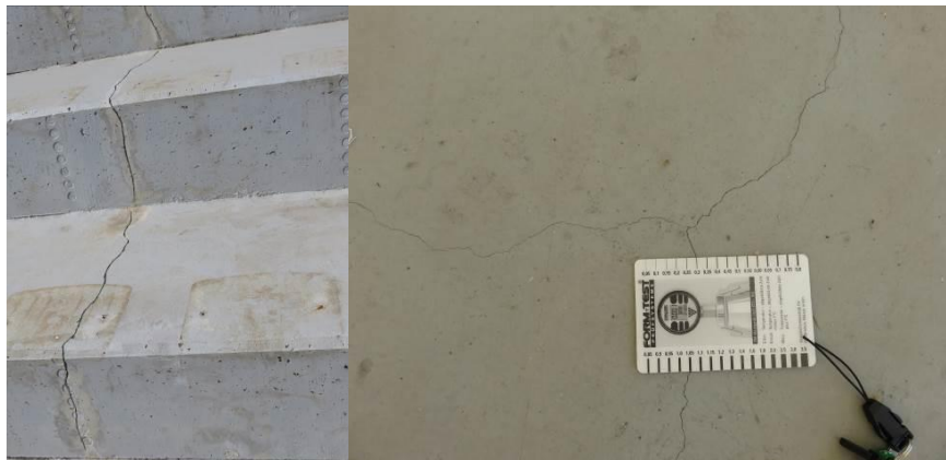
Figure 6: Typical cracks in upper surface
