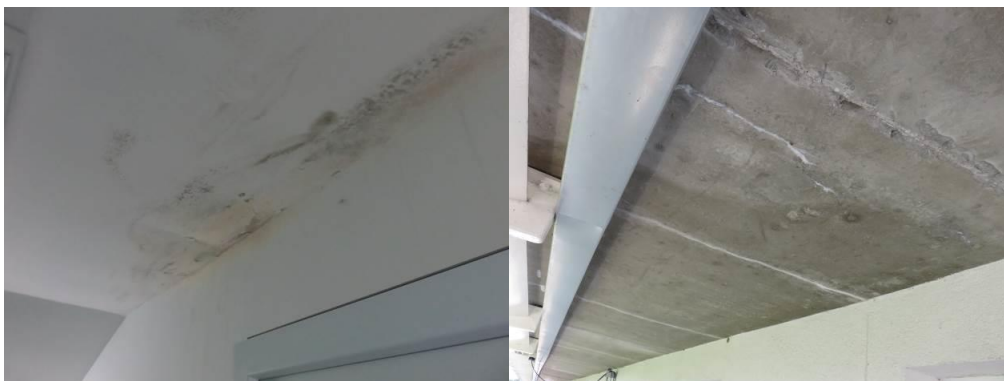
Figure 7: Leakage and lime sediments
