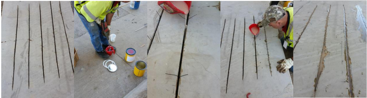
Figure 7: Test installation – from left to right: saw cuts, mixing of epoxy resin, FRP strip introduced and maintained in place using wires, filling of the slot with epoxy resin and result
