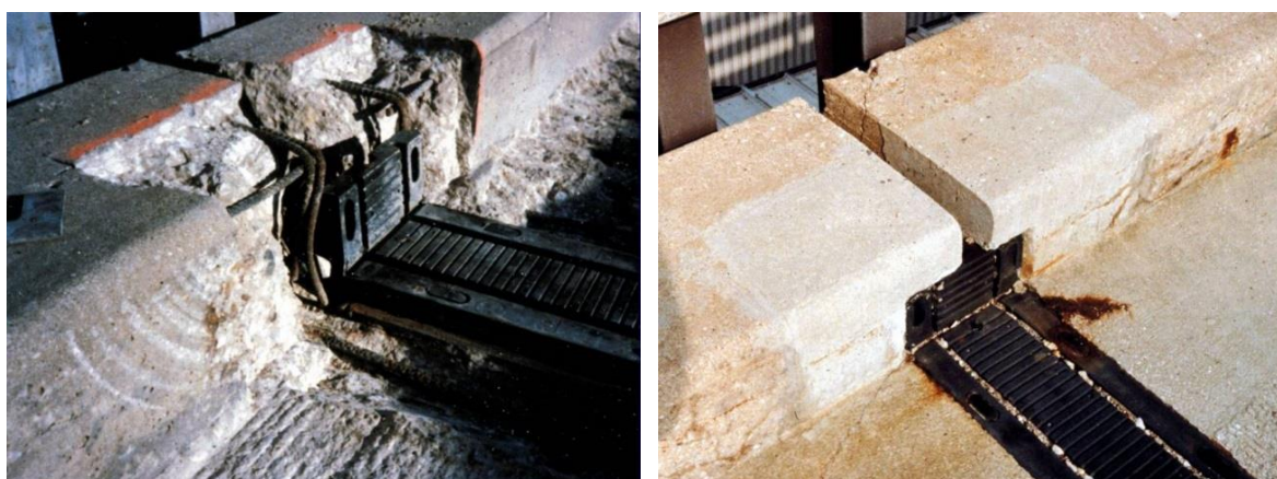
Figure 5: View of patches performed at Argonne bridge. Surface preparation of the concrete to the left, and condition of those repairs 10 years after to the right
