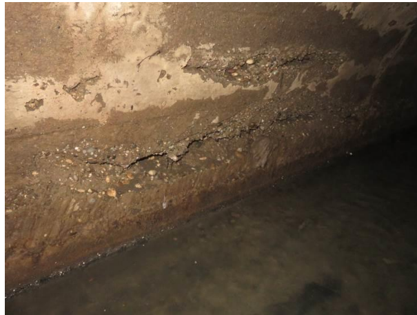
Figure 4: Deterioration of the concrete cladding
