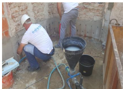
Figure 5: injection into the zone of contact with the ground (STABILCEM, MAPESTOP, LAMPOCEM, MAPE-ANTIQUE INTONACO NHL)
