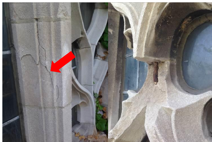
Figure 2 - Cracked and spalled window mullions and rosettes
