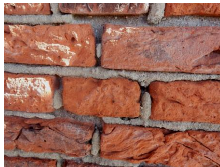
Figure 4: Damage in a trass-lime repointing caused by incomplete hydration of the binding system.
