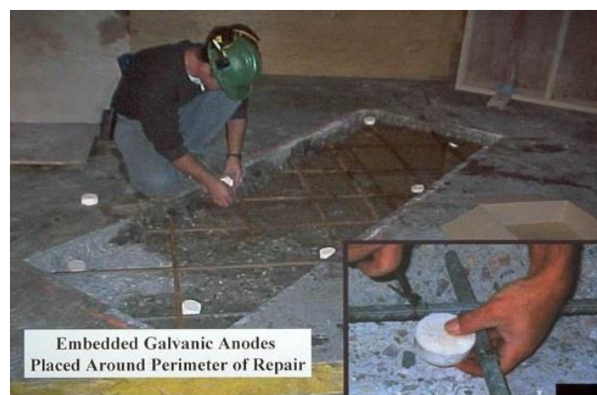
Figure 4: Installation of galvanic corrosion anodes
