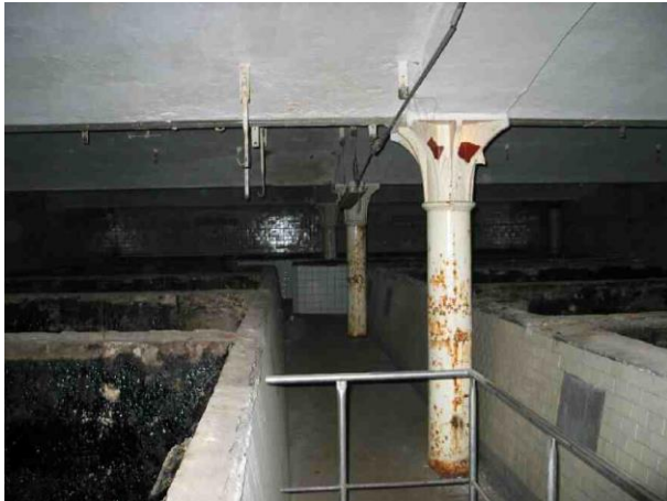
Figure 11: RC reservoirs with cast iron columns
