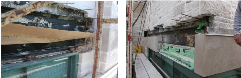
Figure 9 - Repair 6, repairing of steel shelf angles / window lintels at building built in
