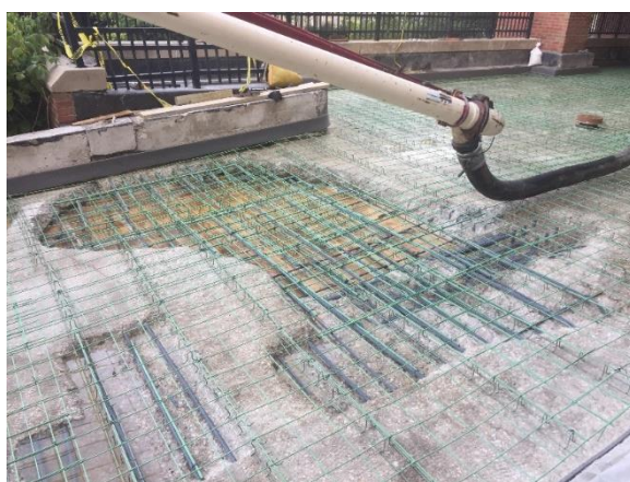
Figure 2: Surface preparation of concrete and coating of reinforcing bars at partial and full depth patches, and installation of new epoxy coated bars for bonded overlay
