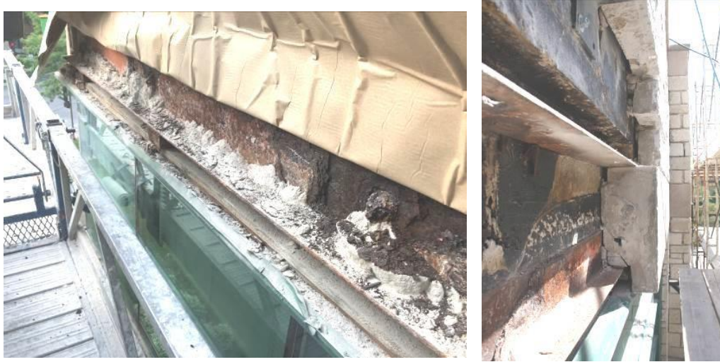
Figure 3 - Severely corroded steel shelf angle and cracked and spalled limestone block due to corrosion
