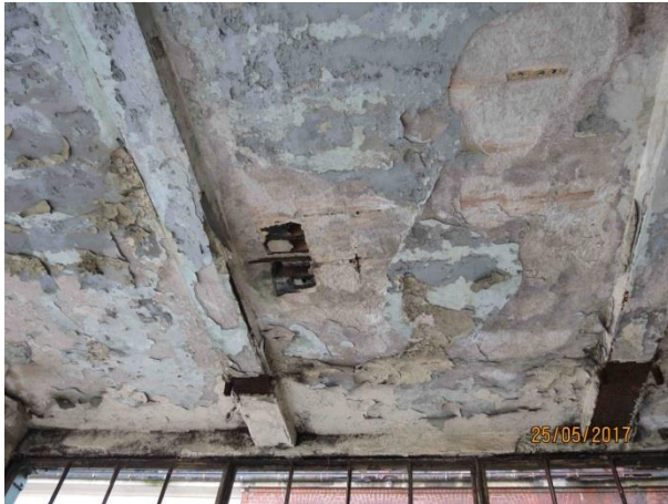
Figure 7: Destruction on Ackerman floors
