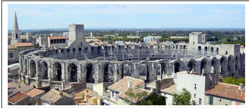
Figure 1: The roman amphitheatre of Arles, before restoration.
