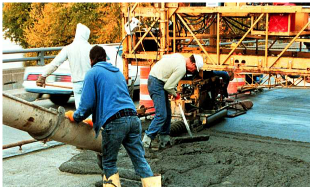
Figure 17: Steel-fibre reinforced concrete overlay instead of traditional bridge insulation
