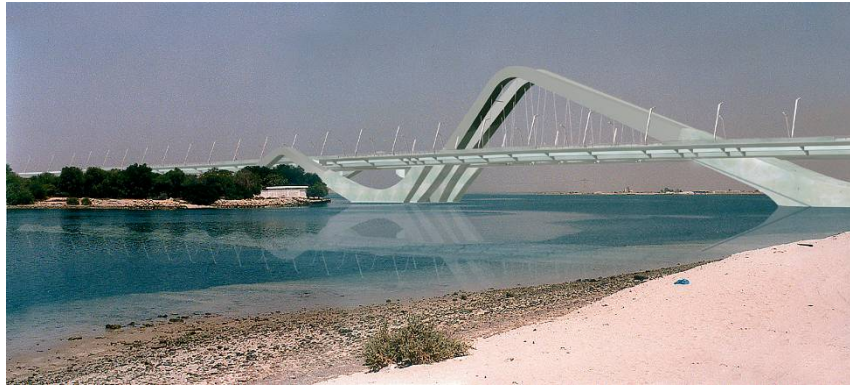
Figure 10: Sheikh Zayed Bridge, Abu Dhabi, selective use of stainless steel reinforcement
