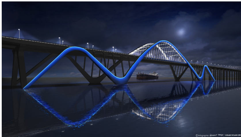
Figure 7: Qatar-Bahrain Causeway at night (rendering by Thomas Lavigne and Christophe Cheron Architects)
